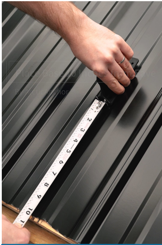
Figure 2 — Setting the eave setback. Measure from the eave edge to the base of the bracket, keeping the tape square to the eave so the setback is identical across the run.
