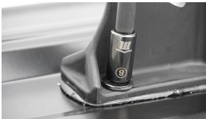
Figure 4 — Seating the washer. Drive until the washer is visibly compressed and the base is pulled flat, then stop.
